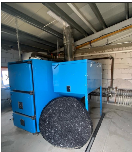
Fig.22 – Centrala termica model MCL BIO R 300
