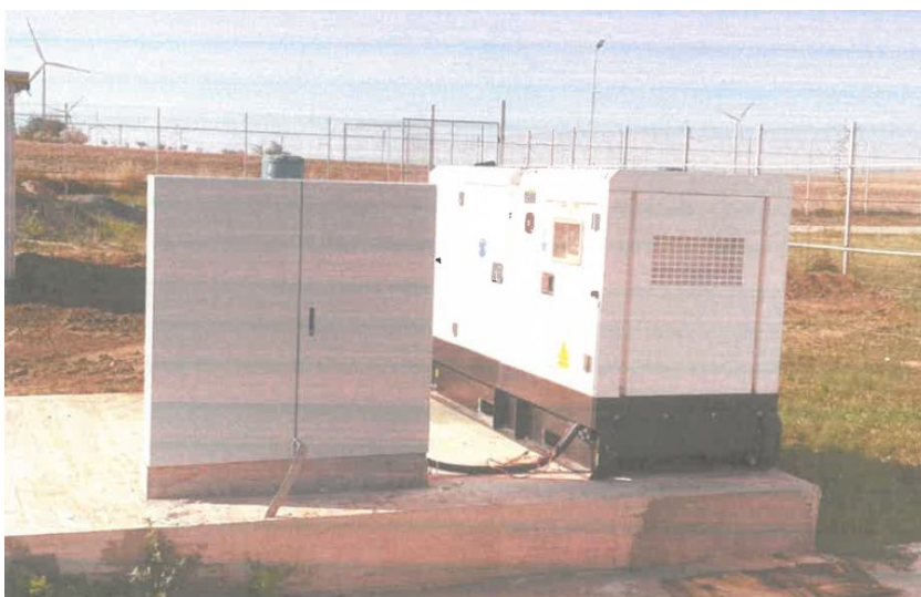
Fig.21 – BMPT si electrogenerator
