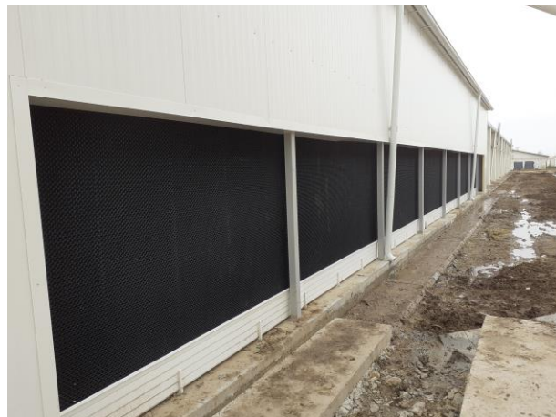
Fig.19 – Sistem de racire tip Pad Cooling (halele H14÷H16)
